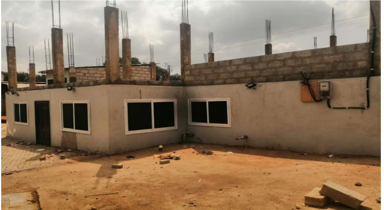
Completed Basement of Clinic at Christian Village
